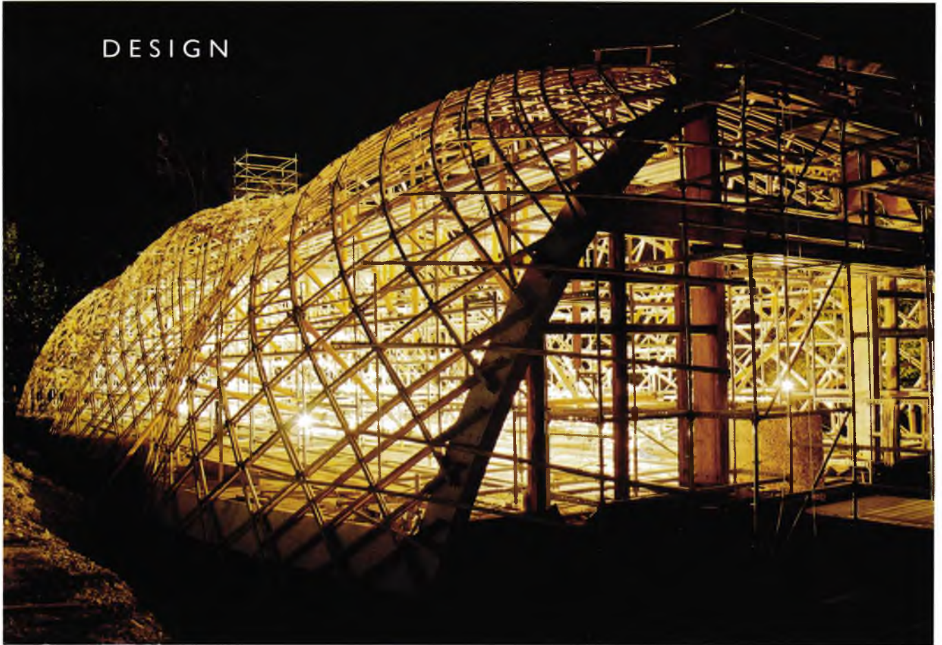
The gridshell framework at night
